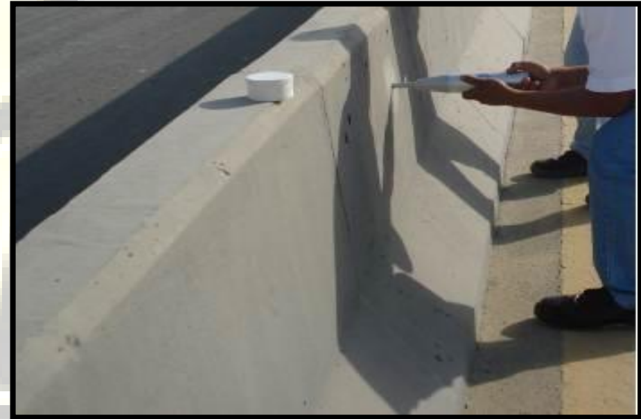
Figure (25): Schmidt hammer test (ASTM C-805)
