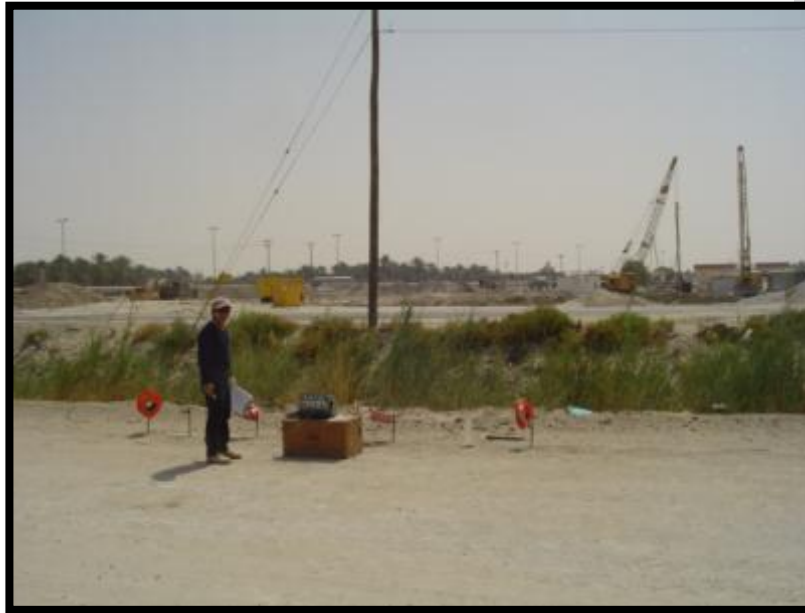
Figure (13): Electrical soil resistivity
