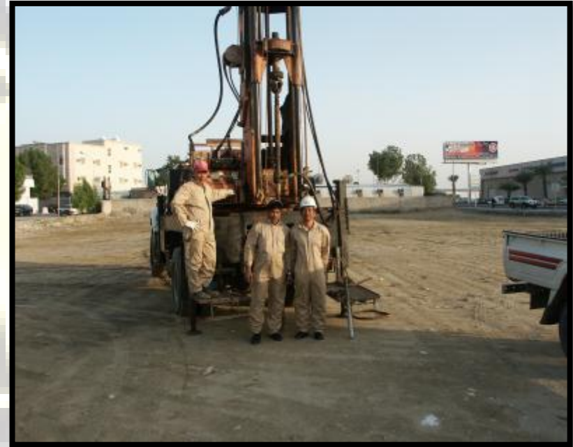
Figure (10): Drilling crew
