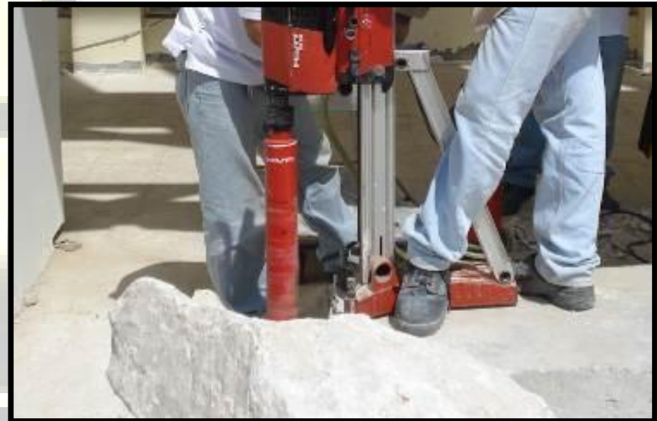
Figure (21): Coring of rock for compressive strength test
