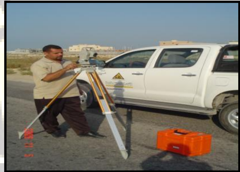
Figure (11): Land Survey
