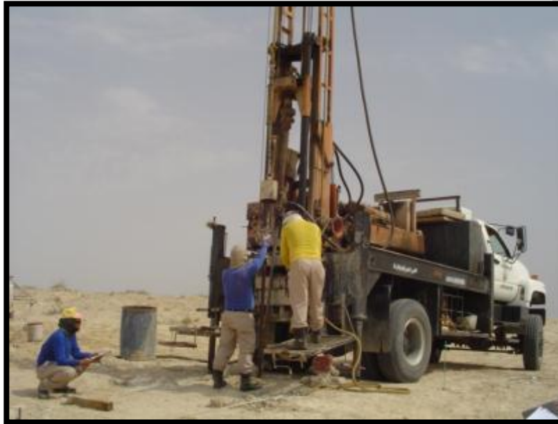
Figure (9): ACKER AD-II rotary drilling rig
